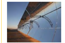
CSP Parabolic Trough
